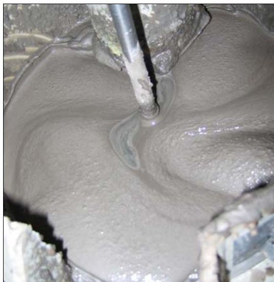
Figure 4.16 Pilot Plant Leach Tank
