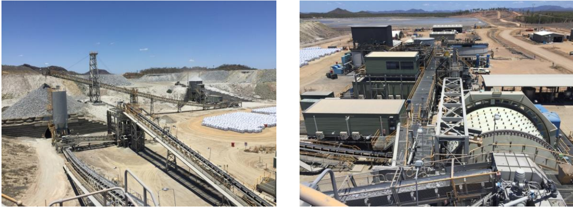
Figure 7 – Primary Crusher, Stockpile, Pebble Crushers, and SAG Mill
