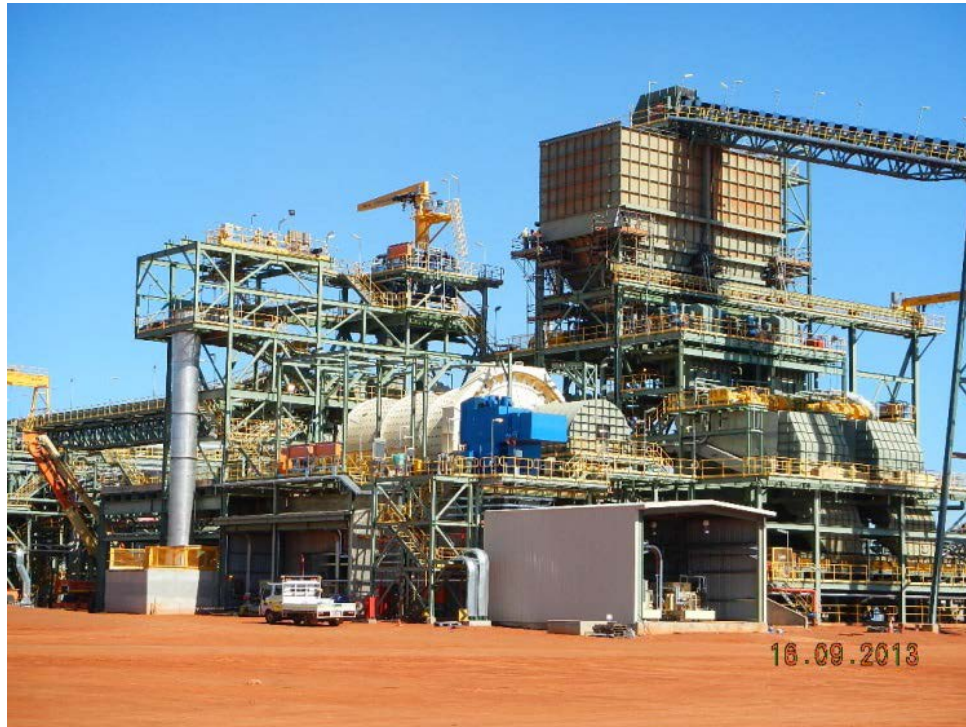
Figure 5 – Tropicana HPGR Screening and Ball Mill Area
