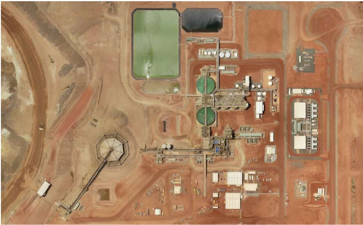
FIG 2 – Gruyere plant aerial photograph.
