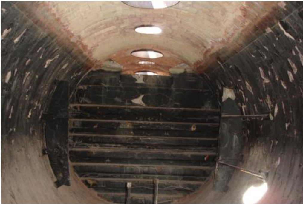
Figure 12 : Copper Pressure Leach Autoclave Internals
